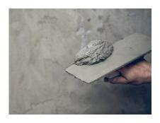
second layer is applied at a maximum thickness of 2-2.5 cm after setting the first layer.
