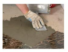
waited until the water layer disappears so that the surface remains moist.
