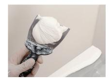
mixture should be rested for 10 minutes before application.
