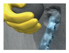
prevent adhesion such as soil, oil, paint, mud and pitch should be cleaned.
