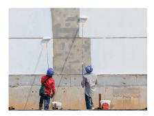
24 hours, the temperature of the environment and the surface to be applied should be minimum +10°C and the surface should not receive precipitation.
