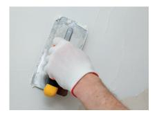
Before application, the surface must be moistened and saturated with water in very hot and windy weather.
