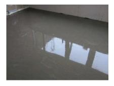
— When the primer is not used, the surface should be cleaned with water for 30 minutes before application. It must be moistened first.
