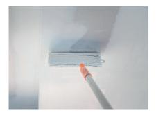
The temperature of the environment and the surface to be applied should be minimum +10°C during the application and for the following 24 hours.
